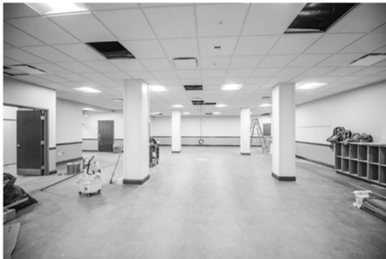
New lecture hall/classroom carved out of the former machine room, February 2021.
